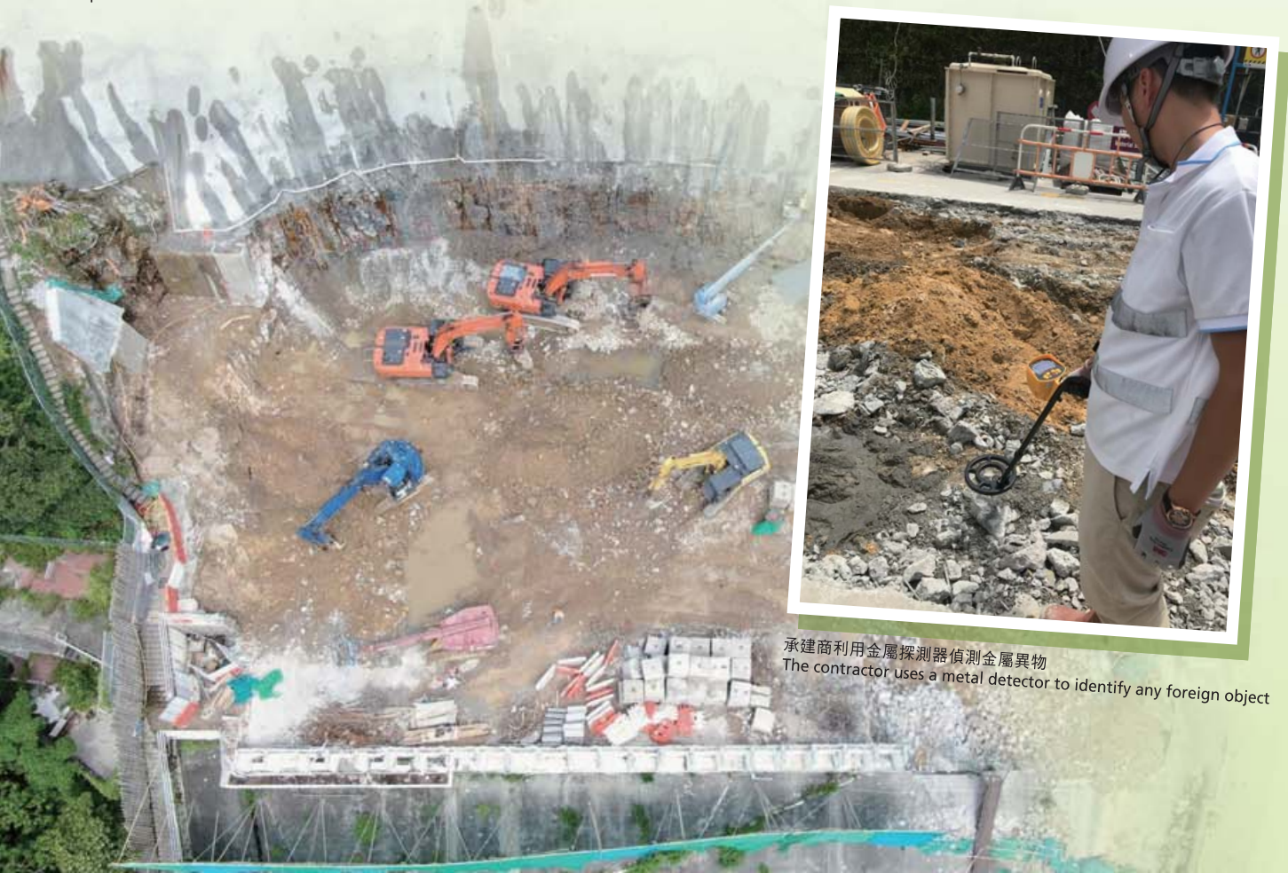
斜坡穩固工程 Slope Stabilization Works
